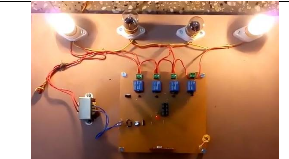
Fig. 4. Remotely Light on using RF Module
